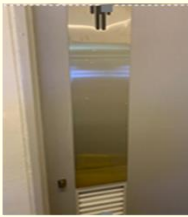
Push doors in toilets and kitchens
